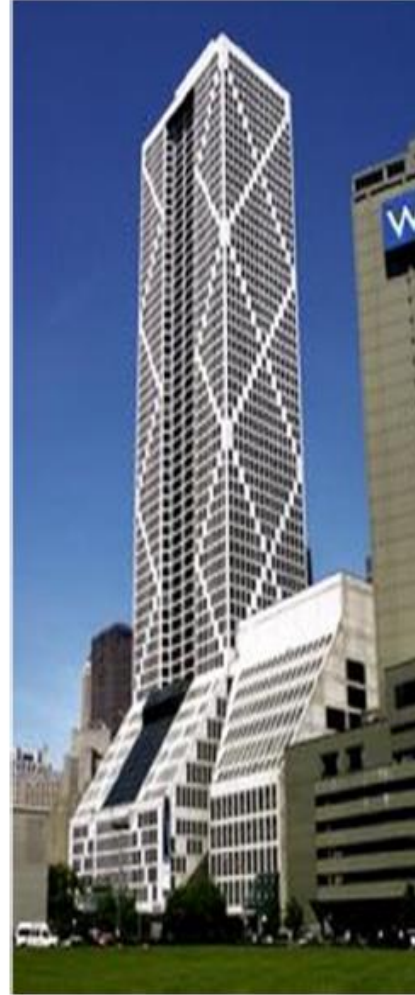
Betonarme, 174 m, 58 katlı, New York
