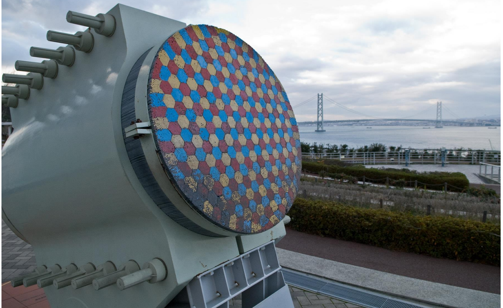
Cable Cross Section of 36,830 Individual Strands with the 4km long bridge in the background
